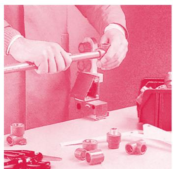
Pipe and fitting are pushed together and become joined in an inseparable manner (do not rotate relative to one another and wait until the cooling time has expired).
